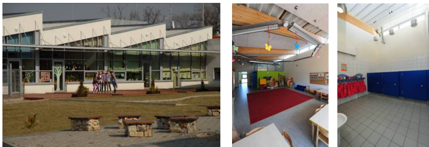
Fig. 1.6 In the preschool area there is a shed roof allowing direct eastern daylight into the rooms and also into half of toilets. a) the shed roof from outside, b) the natural light penetrating the classrooms, c) the restroom illuminated by natural light
