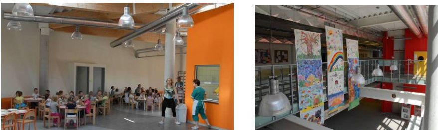
Fig. 1.5 Across the building the construction, electrical and ventilation systems are left visible to show how the building functions. a) Dining area b) Entrance hall
