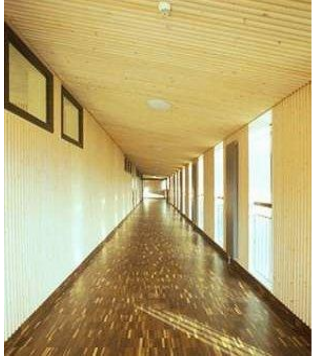
Figure 9: Paul-Moor (ILMASI) School in Garbsten, Germany (2003), Despang Architekten. The mixture of oak and spruce used for timber finishing. Photography: Despang Architekten.
